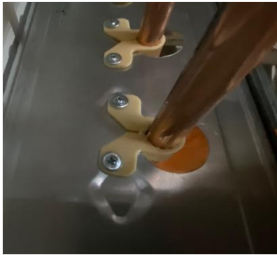
HORIZONTAL_PIPE_BRACING_TO_STUD_WALLS.PNG
