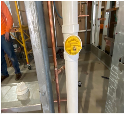
vent_line_plug_clean_outs.jpg
