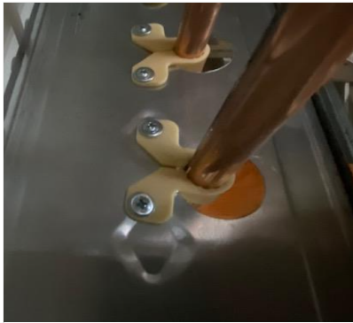
HORIZONTAL_PIPE_BRACING_TO_STUD_WALLS.PNG
