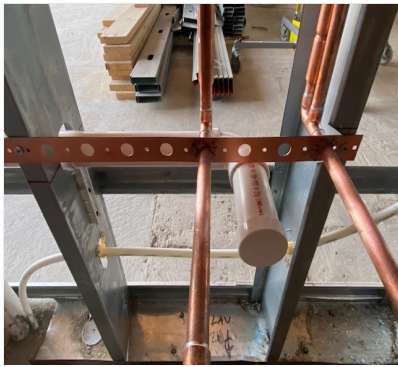
Escutcheon_bracing_at_termination_point.jpg
