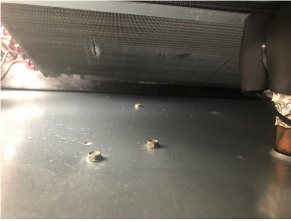
RTU-2 Drain pan
