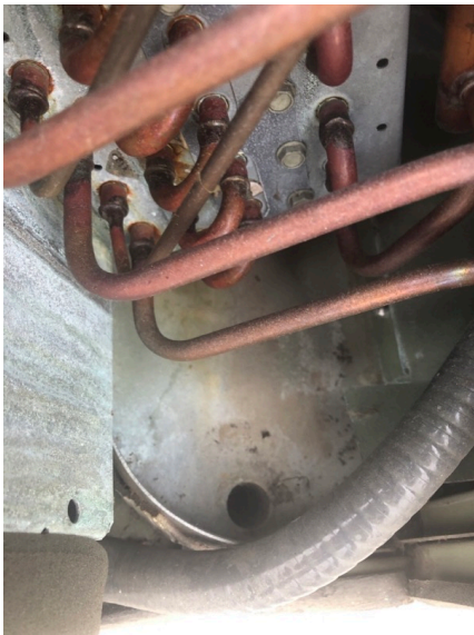
RTU-3 Drain pan
