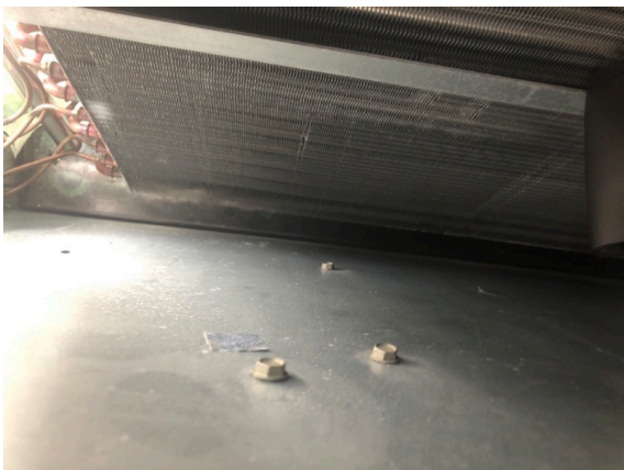
RTU-1 Drain pan
