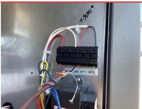
THERMOSTAT WIRING TO DOAS
