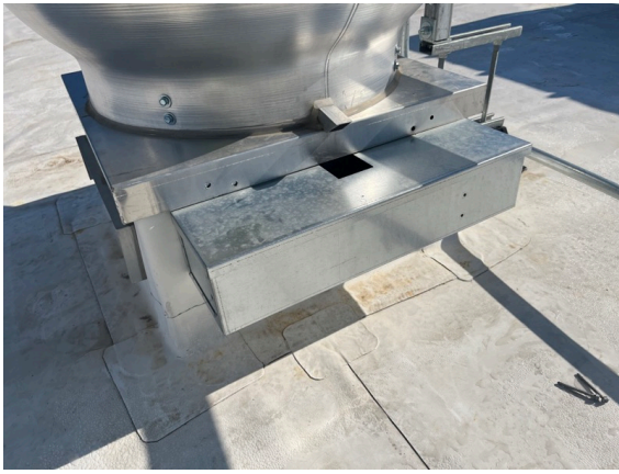
EF-1 Grease cup installed. Fan secured to curb.
