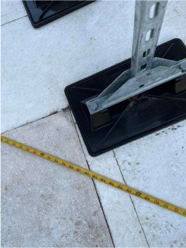
Duct Support Spacing
