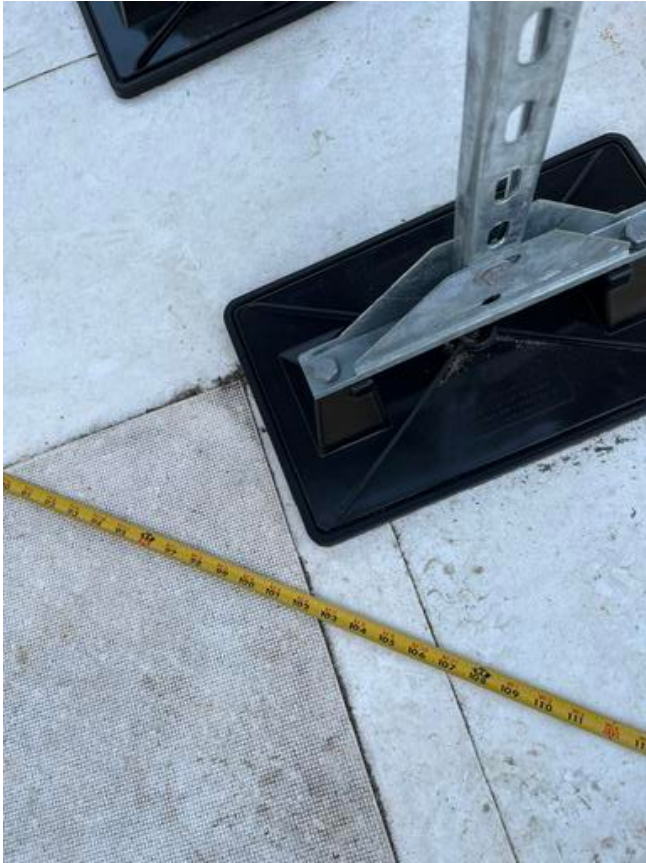
Duct Support Spacing
