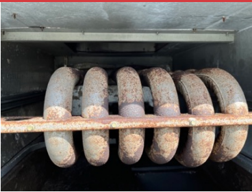
RTU 1 HEAT EXCHANGER TUBES
