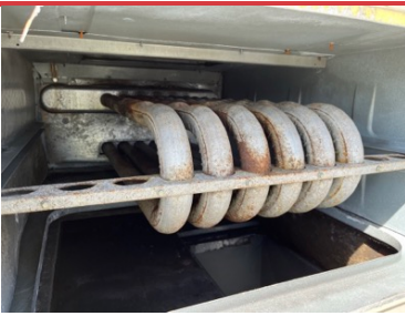
RTU 2 HEAT EXCHANGER TUBES
