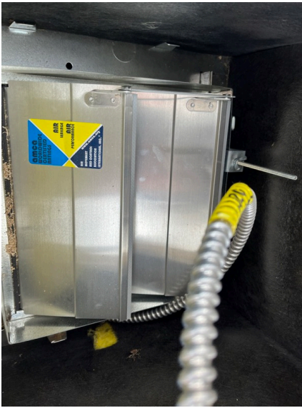
PRV-4 Backdraft damper installed.
