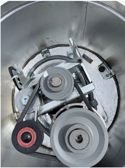
PRV-3 Disconnect installed.
