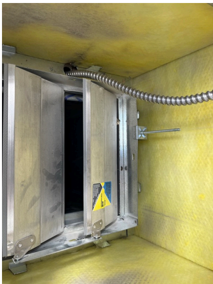
PRV-1 Backdraft damper installed.
