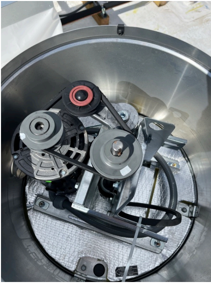
PRV-2 Disconnect installed.
