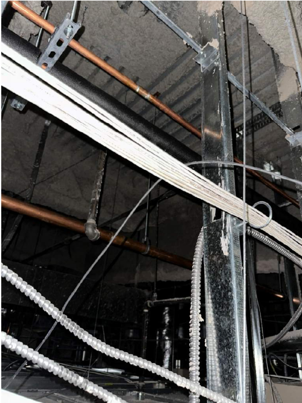
Photograph 3 – Typical view of exposed structural framing
