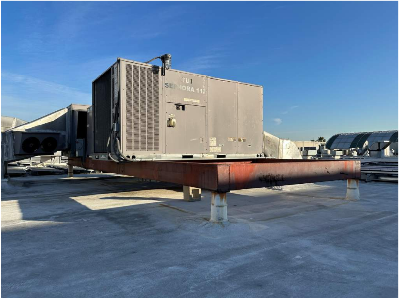
Photograph 5 – Overall view of steel platform above roof
