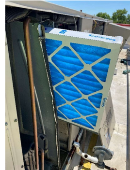
RTU-1 (DINING) CLEAN EVAPORATOR
