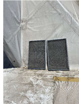
RTU-1 (DINING) CLEAN EVAPORATOR FILTERS
