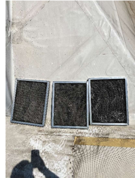
RTU-1 (DINING) CLEAN OUTSIDE AIR FILTERS
