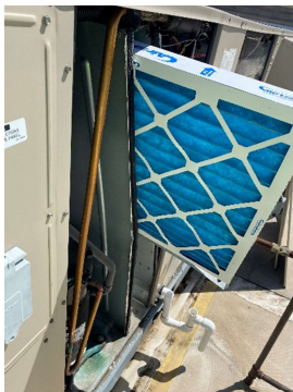
RTU-2 (DINING) DIRTY EVAPORATOR FILTERS
