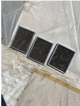
RTU-1 (DINING) DIRTY OUTSIDE AIR FILTERS
