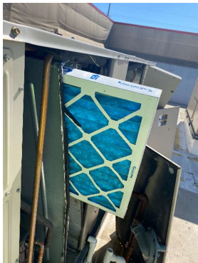
RTU-2 (DINING) DIRTY EVAPORATOR FILTERS
