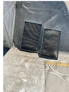
RTU-2 (DINING) CLEAN OUTSIDE AIR FILTERS
