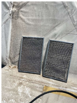
RTU-2 (DINING) DIRTY OUTSIDE AIR FILTERS
