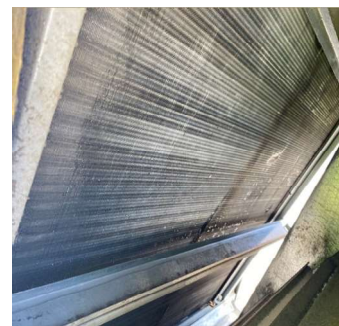
RTU-2 (DINING) CLEAN EVAPORATOR
