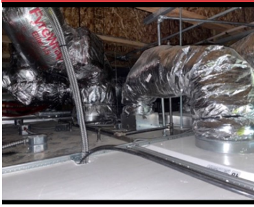
EXTRA EXHAUST FROM HD2 ABOVE CEILING
