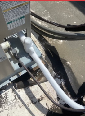
FROZEN LIN ON WALK IN COOLER
