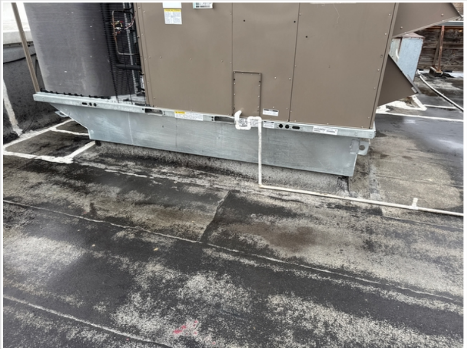
Photo of each unit secured to curb
