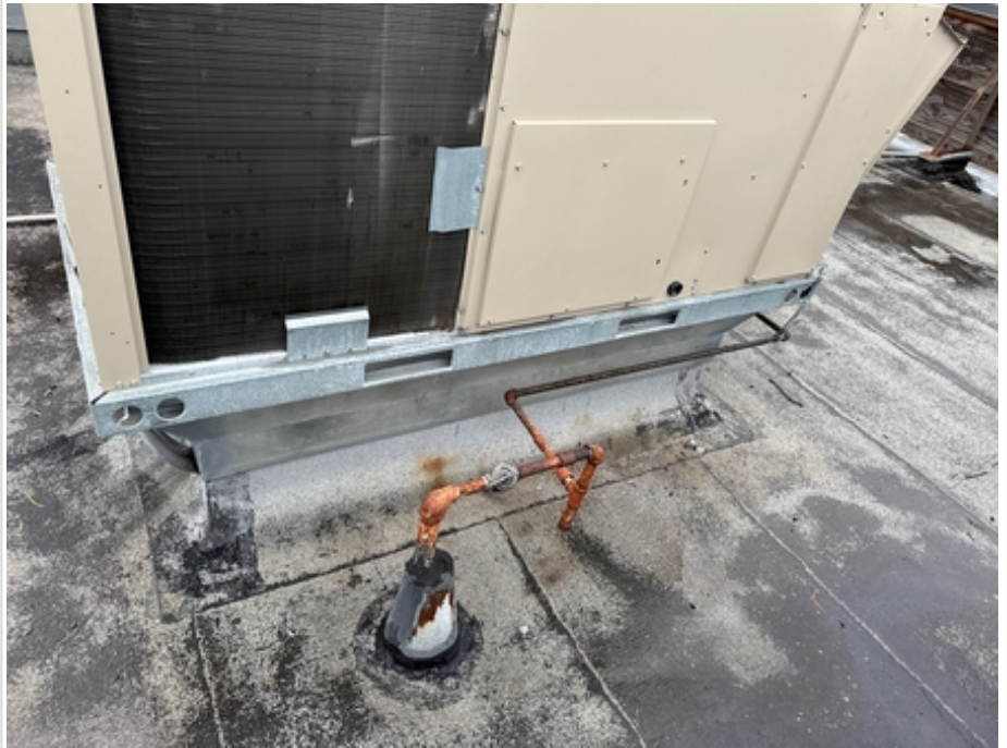
Photo of each unit secured to curb
