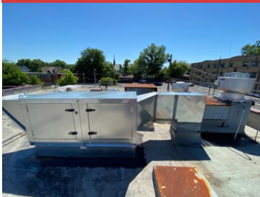
MUA DUCTWORK
