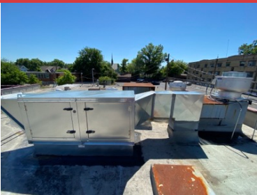
MUA DUCTWORK
