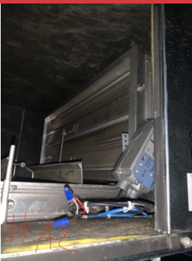
TYPICAL AHU OA AND RETURN DAMPER
