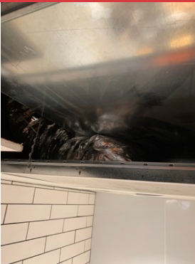
FLEX IS SMASHED DO TO PCU DRIP PAN
