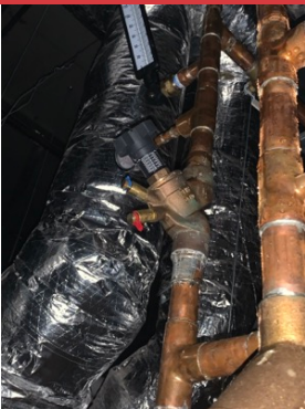
EXAMPLE OF BALANCE VALVE
