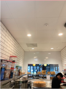
DIFFUSER IN PREP AREA
