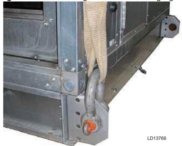
Figure 14 - Correct lifting with base rail
