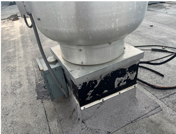
EF-2 No hinge, not secured
