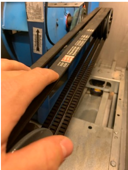
MIDDLE BELT IS BEIT TENSIONED PROPERLY
