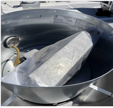
Grease_Cups_Not_Installed 06/11/2024
