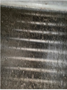
WALK-IN COOLER CLEANED
