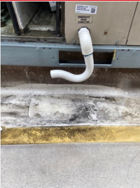
RTU-2 CONDENSATION DRAIN CLEAN
