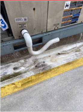
RTU-1 CONDENSATION DRAIN CLEAN
