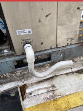
RTU-3 CONDENSATION DRAIN CLEAN
