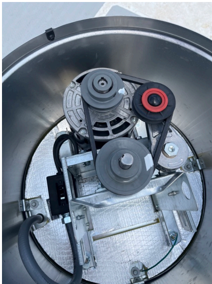
PRV-3 Disconnect installed.
