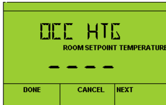
Set occupied heating setpoint [nciTempSetpoints, occupiedHeat]
