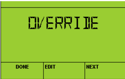
Set overrides for the controller
