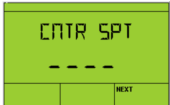
Conventional Wall Module SetPoint Input [nciLogicallyVav, SpcTempSP]
