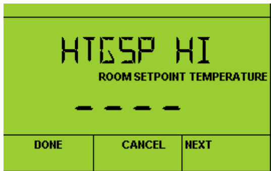
Maximum heating setpoint [nciWallModCom, MaxHtgSetPt]
