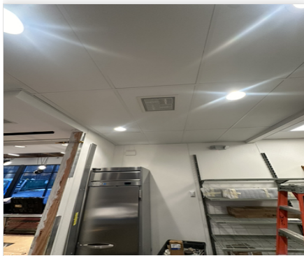
Diffuserwronglocation.. 12/06/2023
