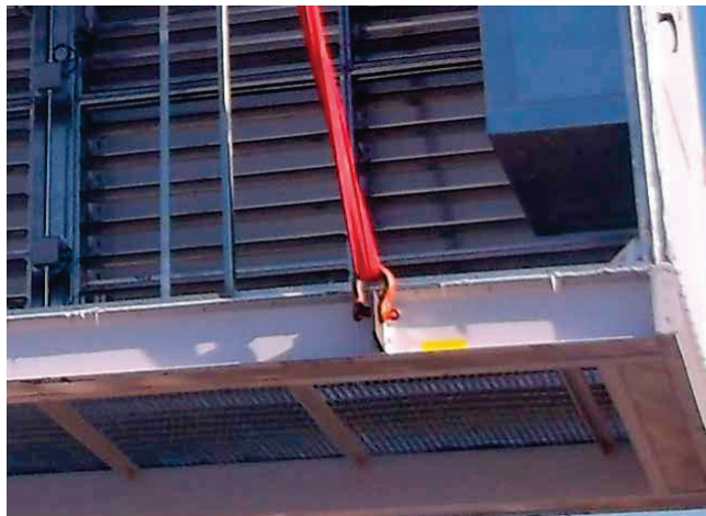
FIGURE 6 - PROPER LIFTING WITH BASE RAIL
