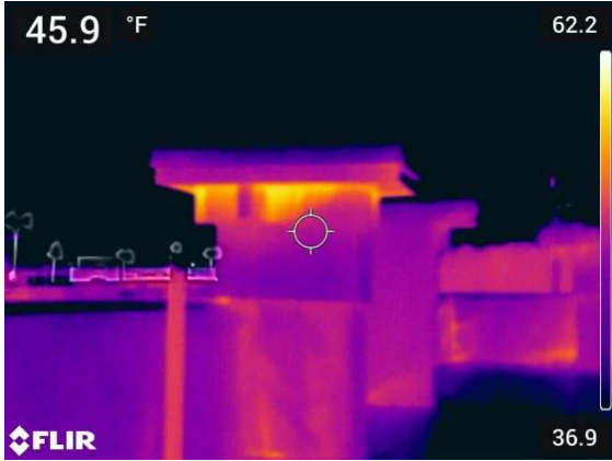
Figure 25. Soffit area from roof
