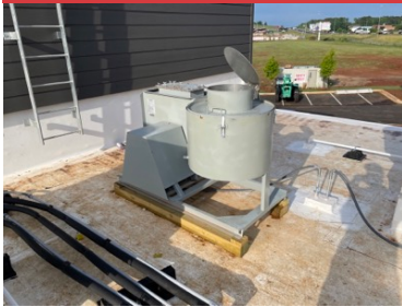
EF1 Connected to HD1A
