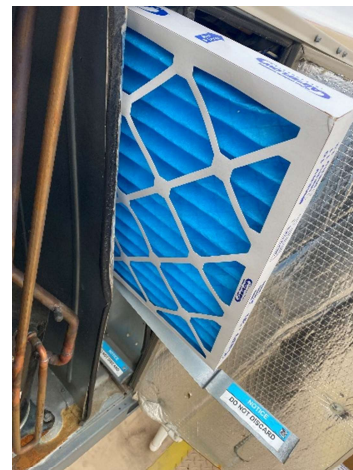
RTU-2 (FRONT KITCHEN/DINING) CLEAN EVAPORATOR FILTERS
