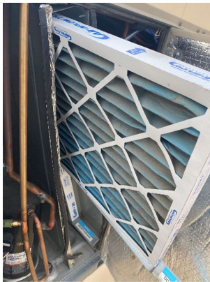
RTU-2 (FRONT KITCHEN/DINING) DIRTY EVAPORATOR FILTERS
