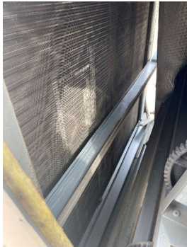
RTU-2 (FRONT KITCHEN/DINING) DIRTY EVAPORATOR
