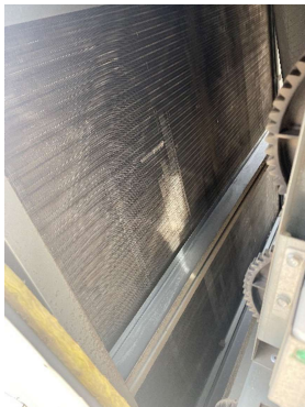
RTU-2 (FRONT KITCHEN/DINING) DIRTY EVAPORATOR
