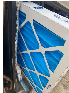
RTU-2 (FRONT KITCHEN/DINING) CLEAN EVAPORATOR FILTERS
