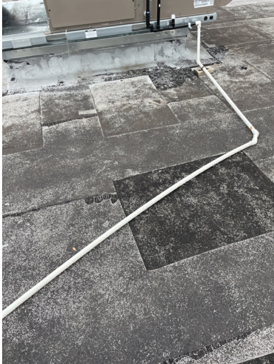
Pictures of RTU Unit Mounting to Roof Curb / Adapter Curb Showing Proper Alignment and Sealing. (2)
