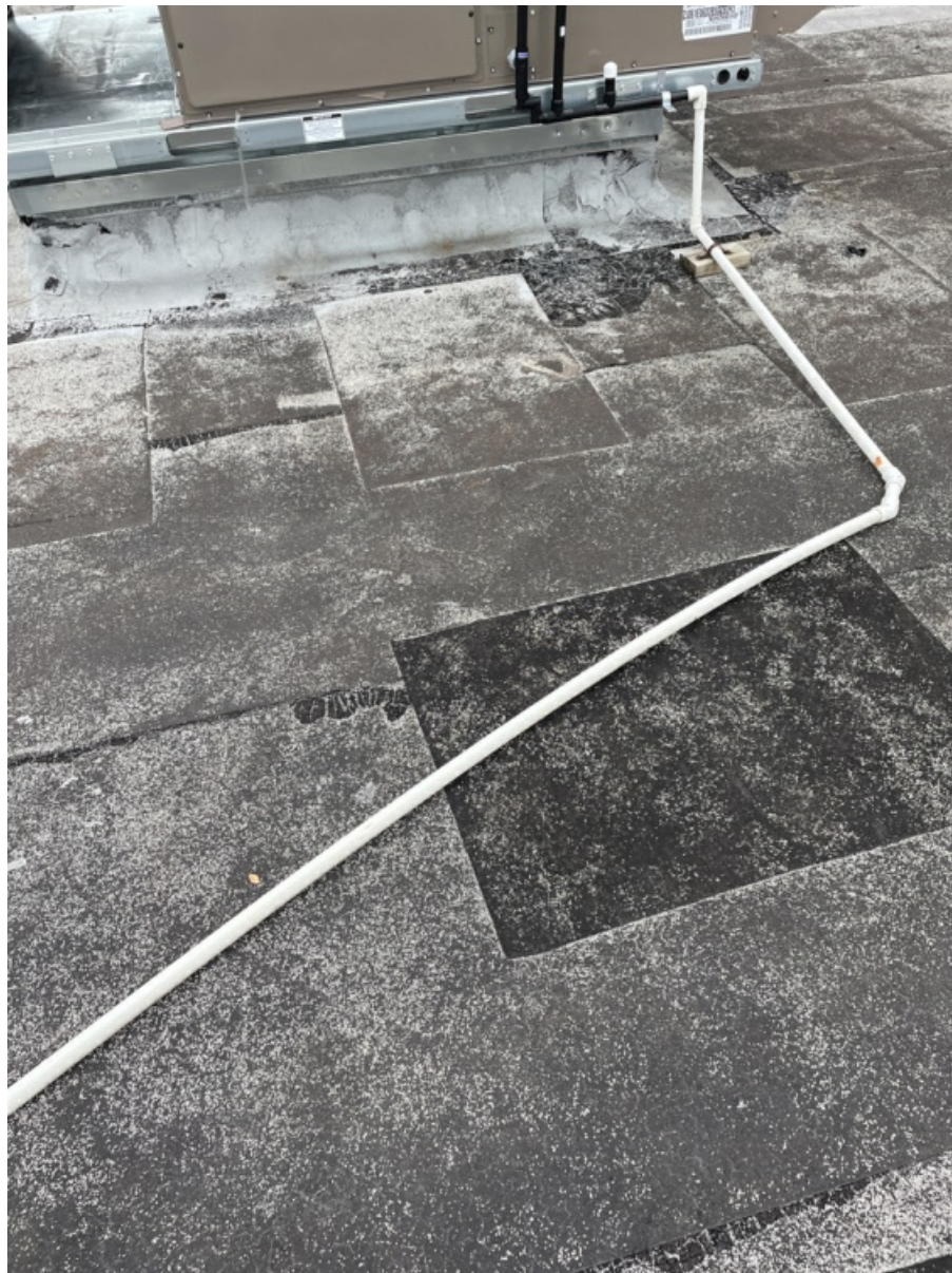
Pictures of RTU Unit Mounting to Roof Curb / Adapter Curb Showing Proper Alignment and Sealing. (1)
