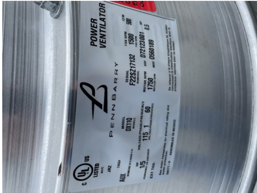
Exhaust Fan Unit Name Plate Photo (5)
