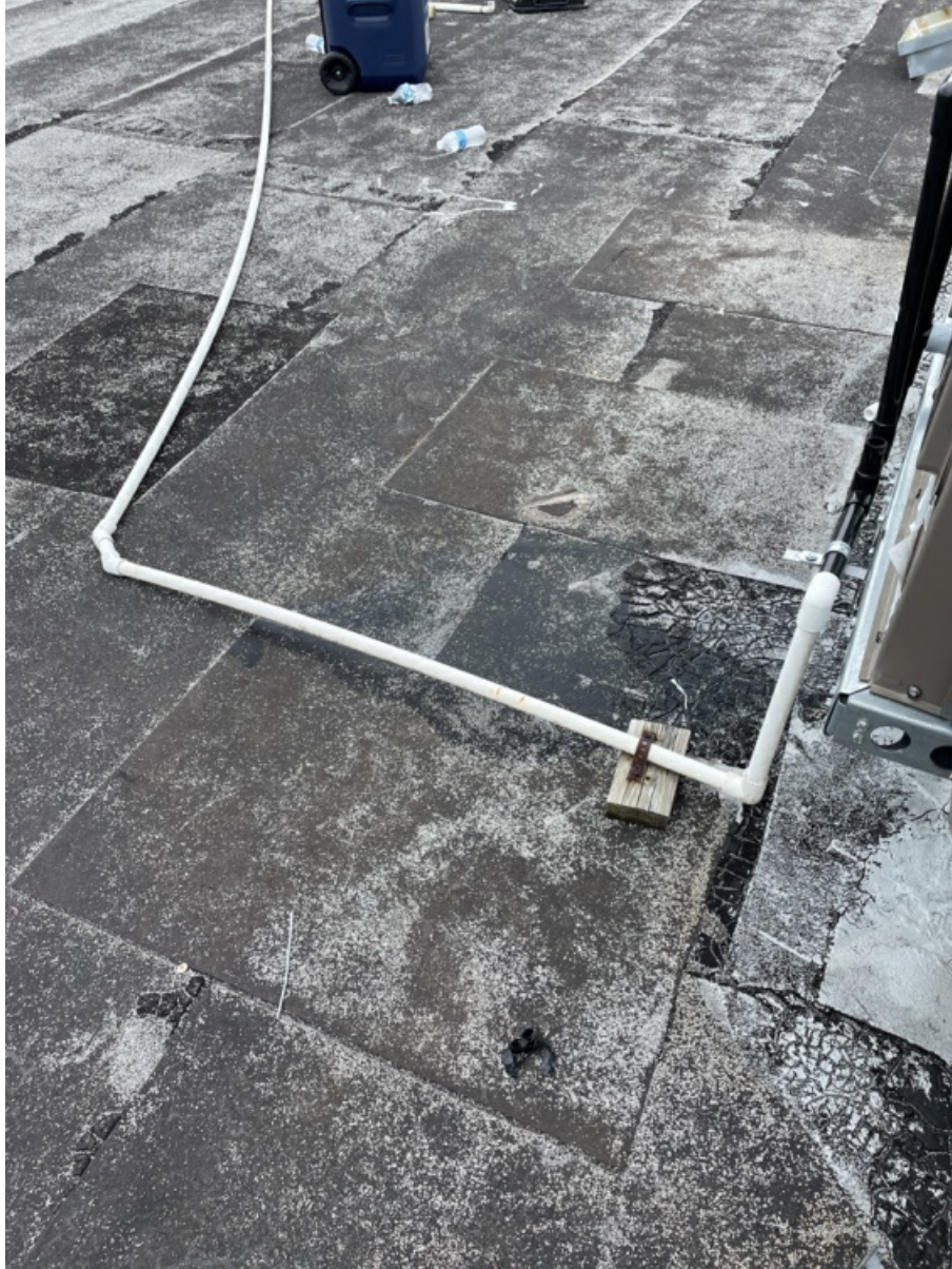
Installed RTU Condensate Drain Photo (1)
