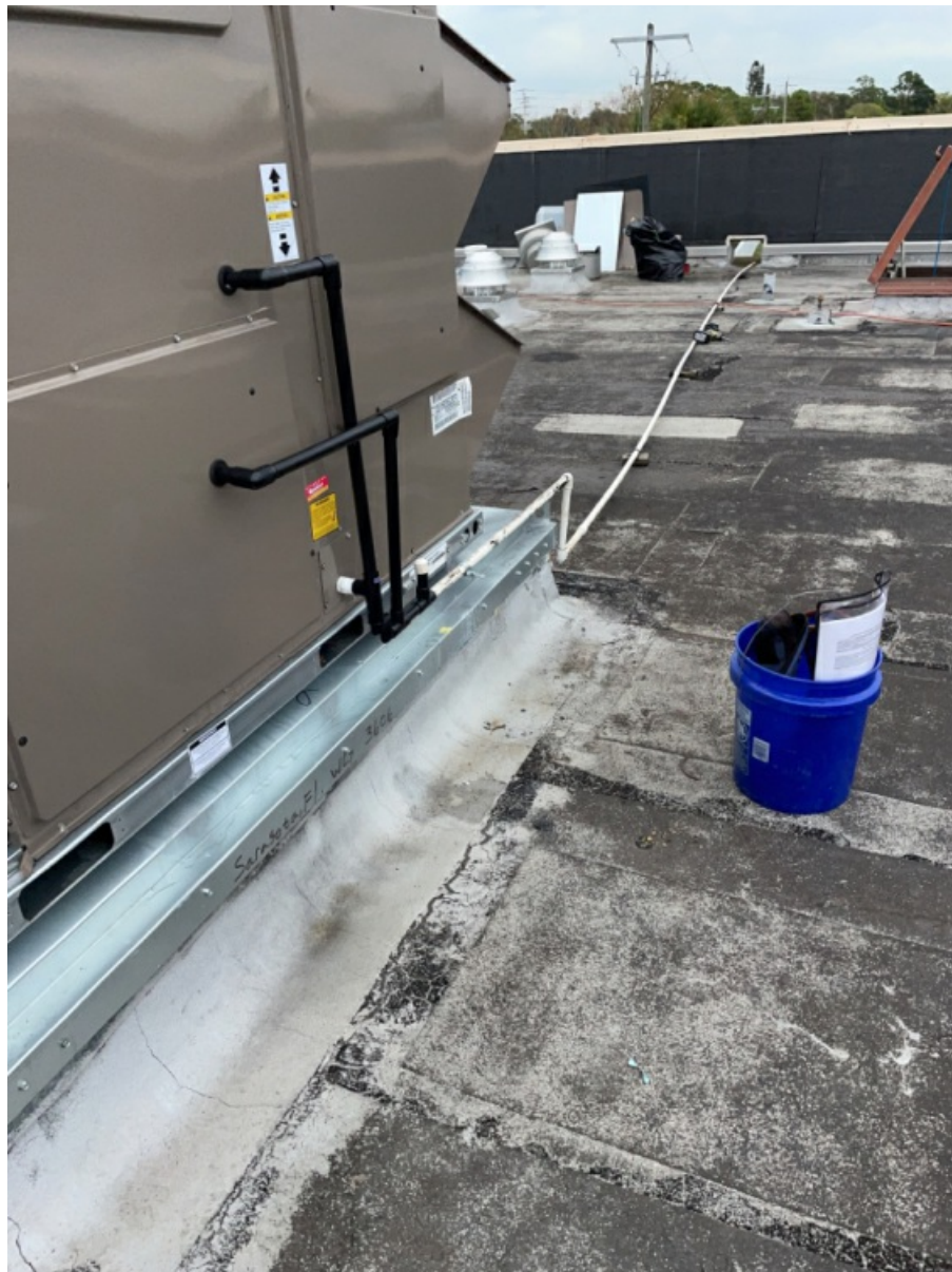
Installed RTU Condensate Drain Photo (1)
