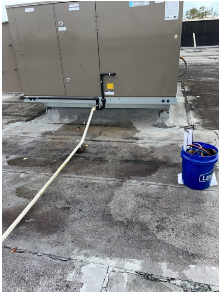
Installed RTU Condensate Drain Photo (1)
