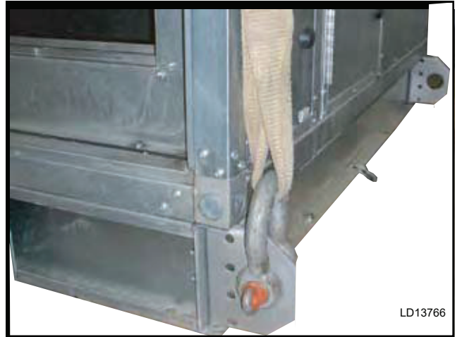
FIG. 1-6 – RECOMMENDED LIFTING WITH BASERAIL
