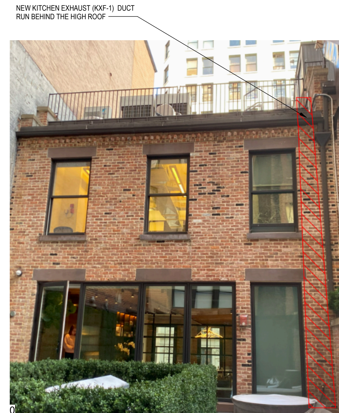
NEW KITCHEN EXHAUST (KXF-1) DUCT RUN BEHIND THE HIGH ROOF
