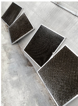
RTU-2 (DINING) DIRTY OUTSIDE AIR FILTERS
