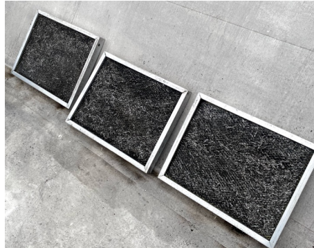
RTU-1 (DINING) CLEAN OUTSIDE AIR FILTERS
