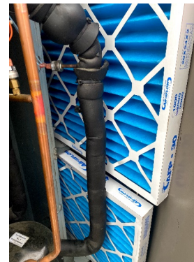
RTU-2 (DINING) CLEAN EVAPORATOR FILTERS
