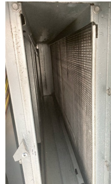
RTU-2 (DINING) CLEAN EVAPORATOR
