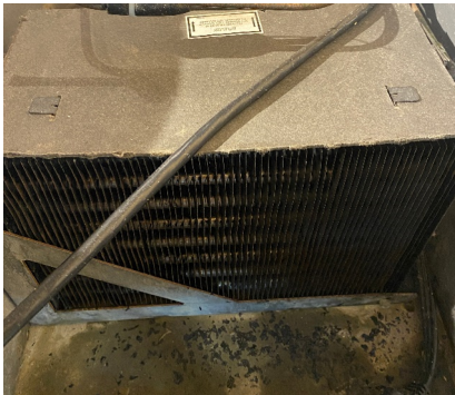
DXC-7 (TOPPING COOLER) DIRTY CONDENSER
