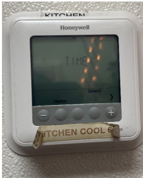
KITCHEN AREA THERMOSTAT UNPROGRAMMABLE
