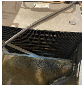
DXC-7 (TOPPING COOLER) CLEAN CONDENSER
