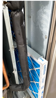
RTU-2 (DINING) CLEAN EVAPORATOR FILTERS
