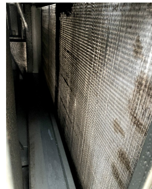
RTU-2 (DINING) CLEAN EVAPORATOR
