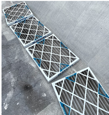
RTU-2 (DINING) DIRTY EVAPORATOR FILTERS
