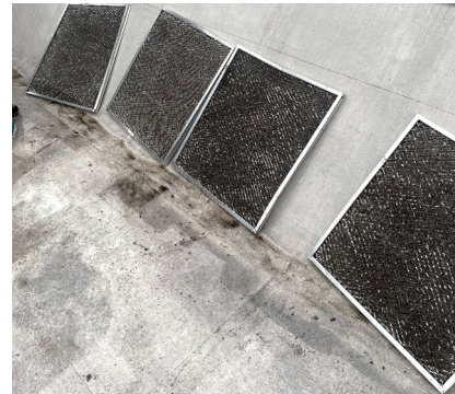
RTU-1 (DINING) CLEAN EVAPORATOR FILTERS
