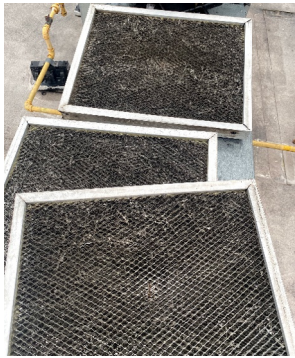
RTU-1 (DINING) DIRTY OUTSIDE AIR FILTERS
