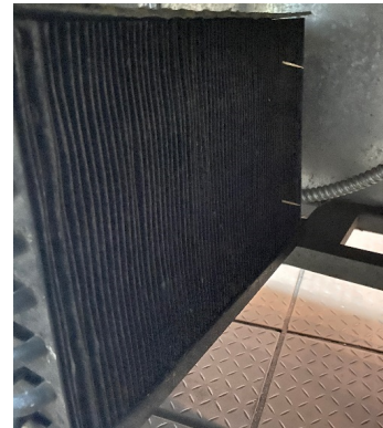
DXC-7 (TOPPING COOLER) CLEAN CONDENSER
