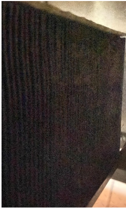
DXC-7 (TOPPING COOLER) DIRTY CONDENSER
