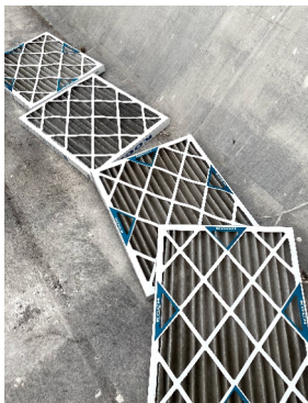
RTU-2 (DINING) DIRTY EVAPORATOR FILTERS
