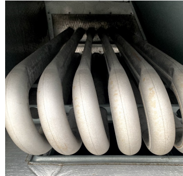
RTU-2 (DINING) BURNER TUBE INSPECTION
