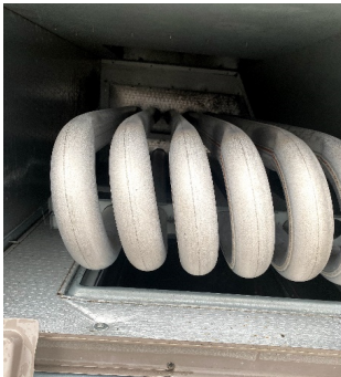
RTU-1 (DINING) BURNER TUBE INSPECTION
