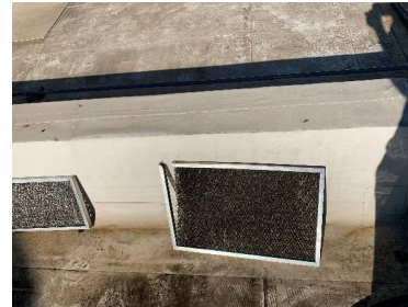
RTU-1 (DINING) CLEAN EVAPORATOR FILTERS
