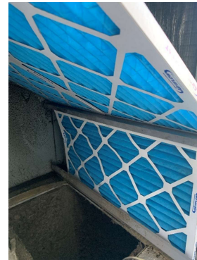
RTU-1 (DINING) CLEAN EVAPORATOR FILTERS
