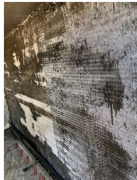
RTU-4 (KITCHEN) CLEAN EVAPORATOR
