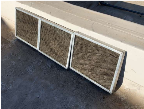
RTU-1 (DINING) DIRTY OUTSIDE AIR FILTERS
