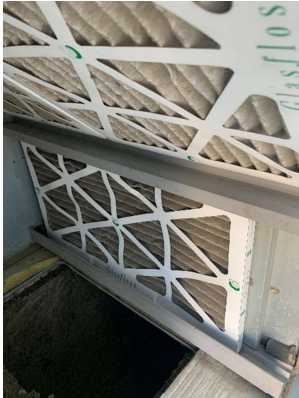
FURNACE DIRTY EVAPORATOR FILTERS
