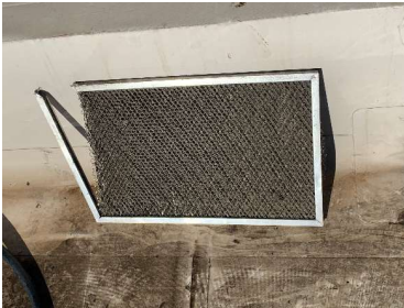
RTU-1 (DINING) DIRTY EVAPORATOR FILTERS
