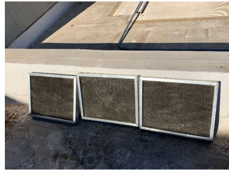
RTU-1 (DINING) CLEAN OUTSIDE AIR FILTERS
