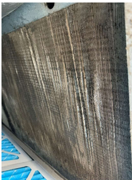
RTU-3 (DINING/ORDERING) DIRTY EVAPORATOR
