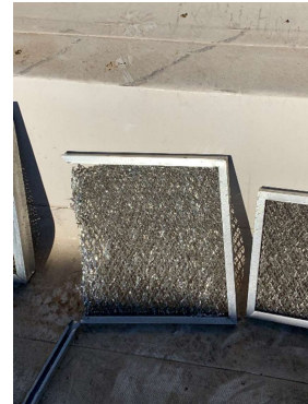
RTU-2 (DINING) CLEAN OUTSIDE AIR FILTERS
