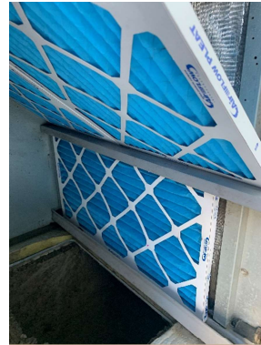
FURNACE CLEAN EVAPORATOR FILTERS
