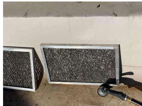
RTU-2 (DINING) CLEAN OUTSIDE AIR FILTERS
