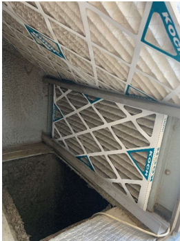
RTU-3 (DINING/ORDERING) DIRTY EVAPORATOR FILTERS
