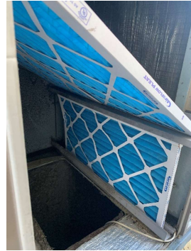
RTU-3 (DINING/ORDERING) CLEAN EVAPORATOR FILTERS
