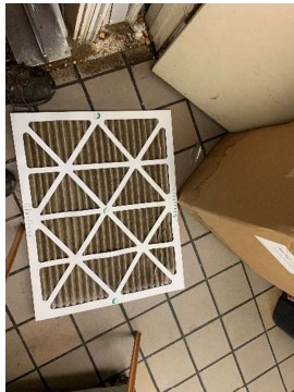
FURNACE DIRTY EVAPORATOR FILTERS
