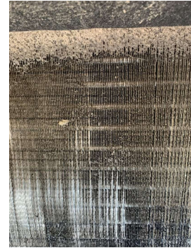
RTU-2 (DINING) CLEAN EVAPORATOR
