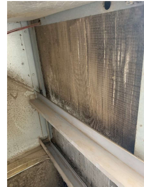
RTU-3 (DINING/ORDERING) CLEAN EVAPORATOR
