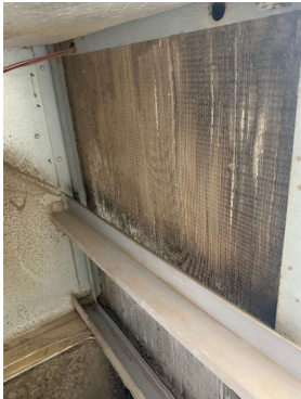
RTU-3 (DINING/ORDERING) DIRTY EVAPORATOR
