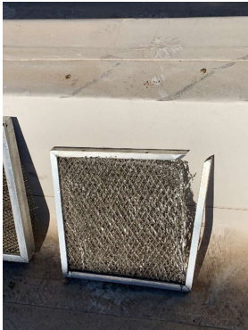
RTU-2 (DINING) DIRTY OUTSIDE AIR FILTERS
