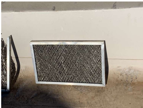
RTU-2 (DINING) DIRTY OUTSIDE AIR FILTERS
