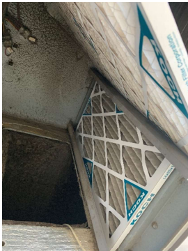
RTU-1 (DINING) DIRTY EVAPORATOR FILTERS
