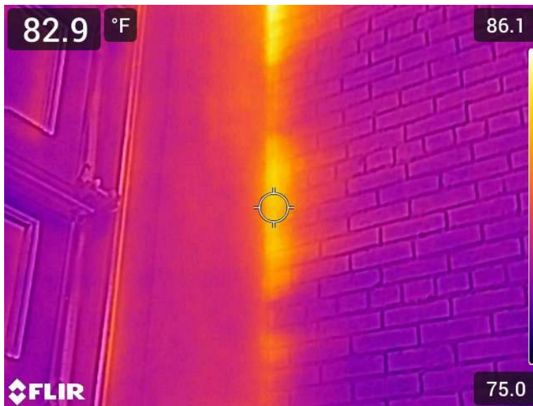
Figure 4. Near garage door on East side
