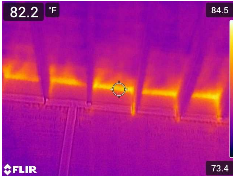
Figure 1. North side of the empty tenant space
