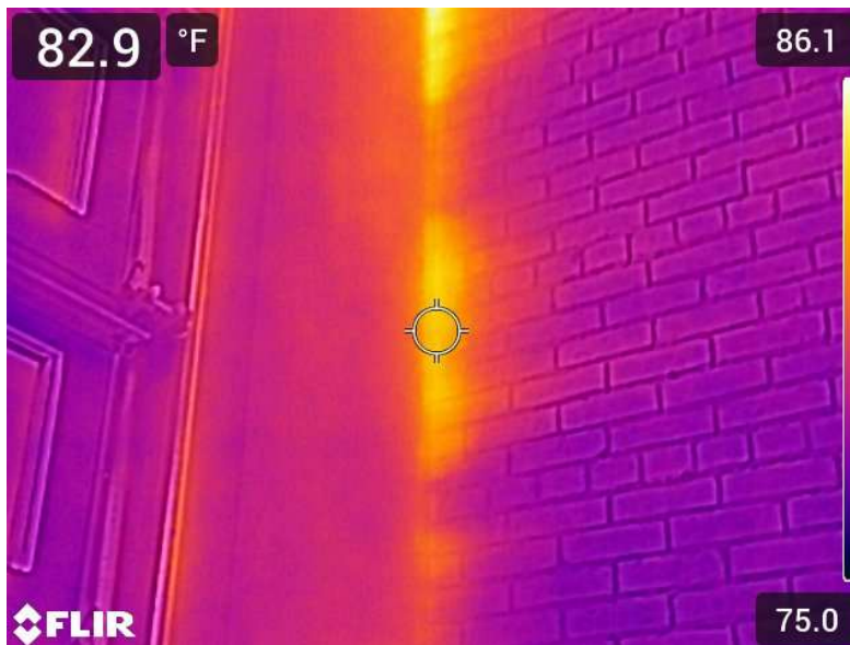
Figure 4. Near garage door on East side
