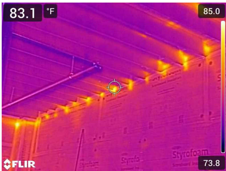
Figure 2. North side of the empty tenant space
