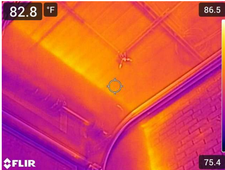
Figure 3. Near garage door on East side
