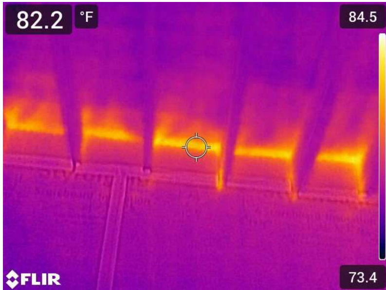
Figure 1. North side of the empty tenant space
