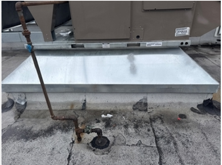
Photo of each unit secured to curb
