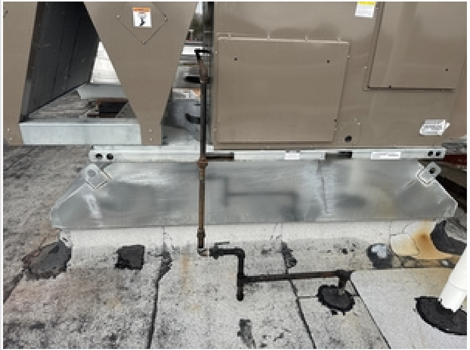
Photo of each unit secured to curb
