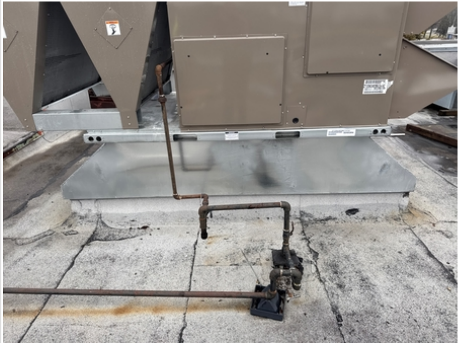
Photo of each unit secured to curb
