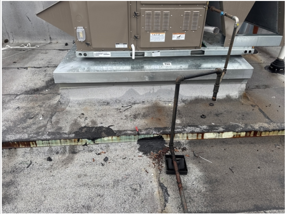
Photo of each unit secured to curb
