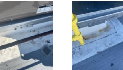
If Seismic Adapter Clips Furnished and Installed on RTU, take Photo
