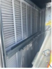
Installed RTU Air Filter Photo
