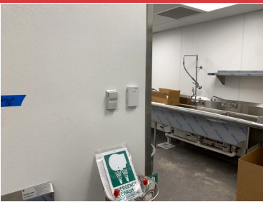
RTU-2 SENSOR LOCATION
