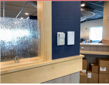
RTU-1 SENSOR LOCATION
