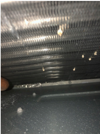
RTU-1 Drain pan
