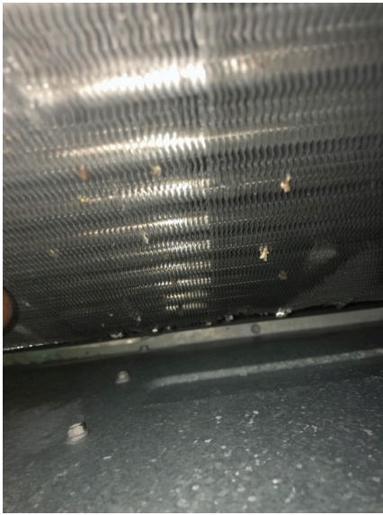
RTU-2 Drain pan
