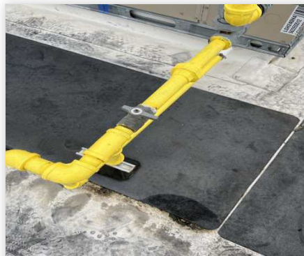
RTU_1GASVALVESHUTCARM.. 10/25/2023
