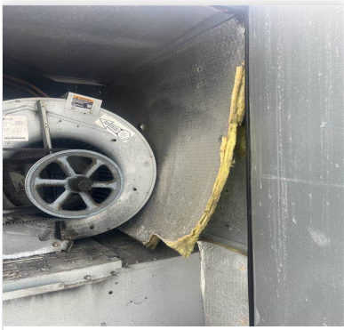
RTU_2_Insulation_Loose 06/20/2024
