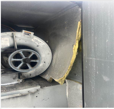
RTU_2_Insulation_Loose 06/20/2024
