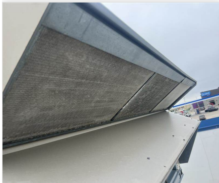
RTU_2_OA_FILTERS 06/20/2024
