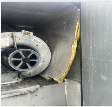
RTU_2_Insulation_Loose 06/20/2024
