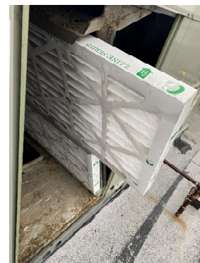
RTU-1 (DINING) CLEAN EVAPORATOR FILTERS
