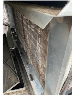
RTU-2 (FRONT KITCHEN/DINING) CLEAN EVAPORATOR
