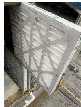
RTU-1 (DINING) CLEAN EVAPORATOR FILTERS
