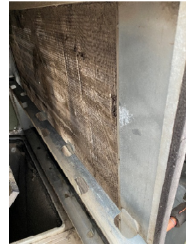
RTU-2 (FRONT KITCHEN/DINING) CLEAN EVAPORATOR
