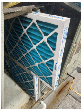
RTU-1 (DINING) DIRTY EVAPORATOR FILTERS
