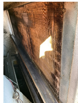
RTU-3 (DINING/RR) CLEAN EVAPORATOR
