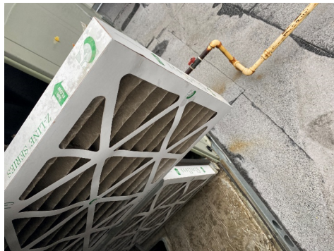
RTU-3 (DINING/RR) DIRTY EVAPORATOR FILTERS
