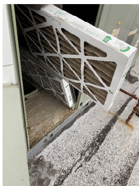
RTU-1 (DINING) DIRTY EVAPORATOR FILTERS
