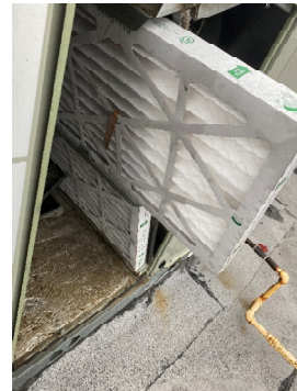
RTU-3 (DINING/RR) CLEAN EVAPORATOR FILTERS
