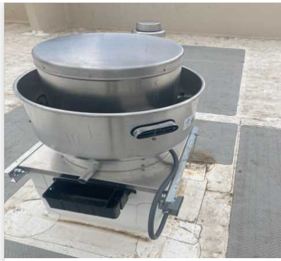
grease_cups_installed...
