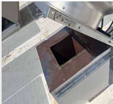
tension_wire_missing....
