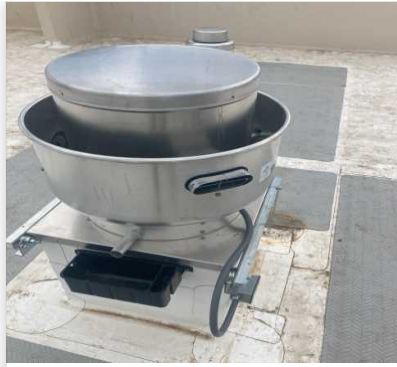
grease_cups_installed...
