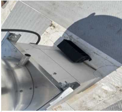
grease_cup_not_instal...
